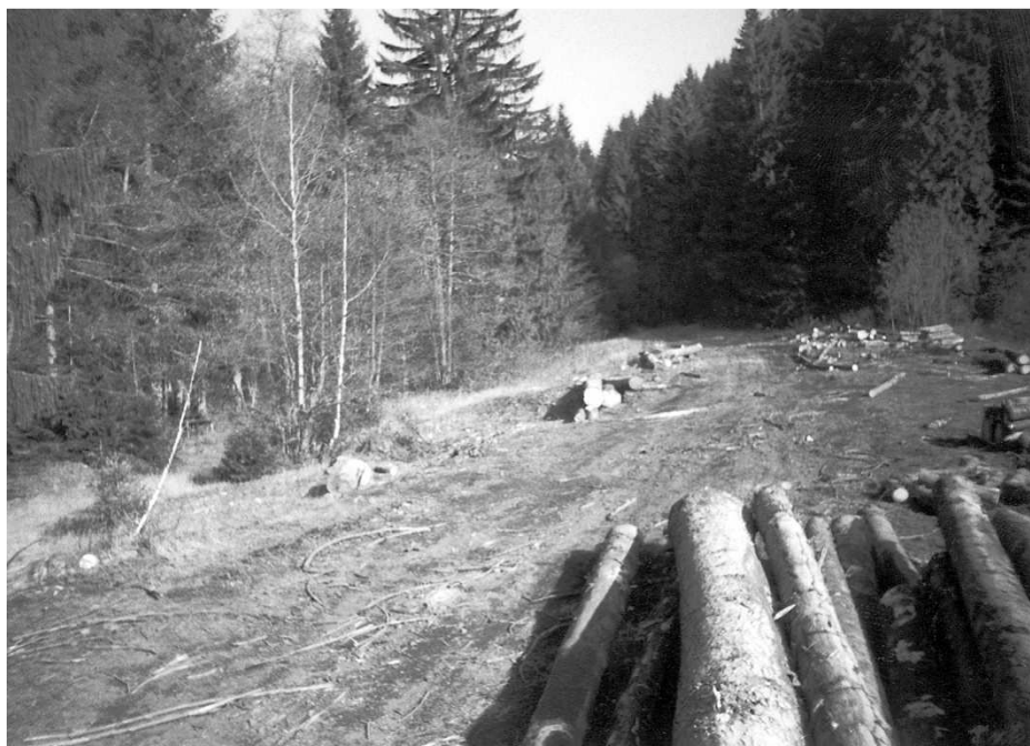
Fig. 9. reinforcement of forest roads in Peklo valley by material from slag-heaps.
