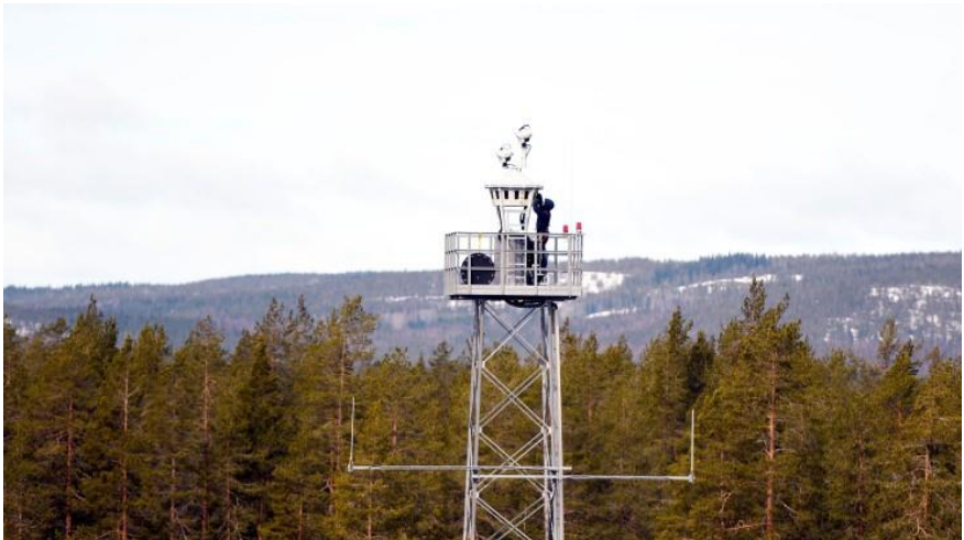
Fig.2 Camera system for remote control tower Source: [11]
